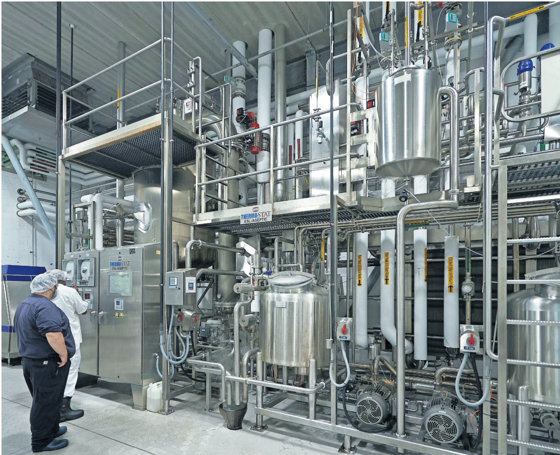
An aseptic milk pasteurizer at Byrne. CHUCK WAINWRIGHT
